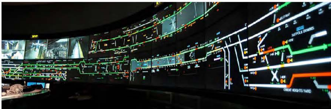
Figure 6: Massachusetts Bay Transit Authority Control Room
