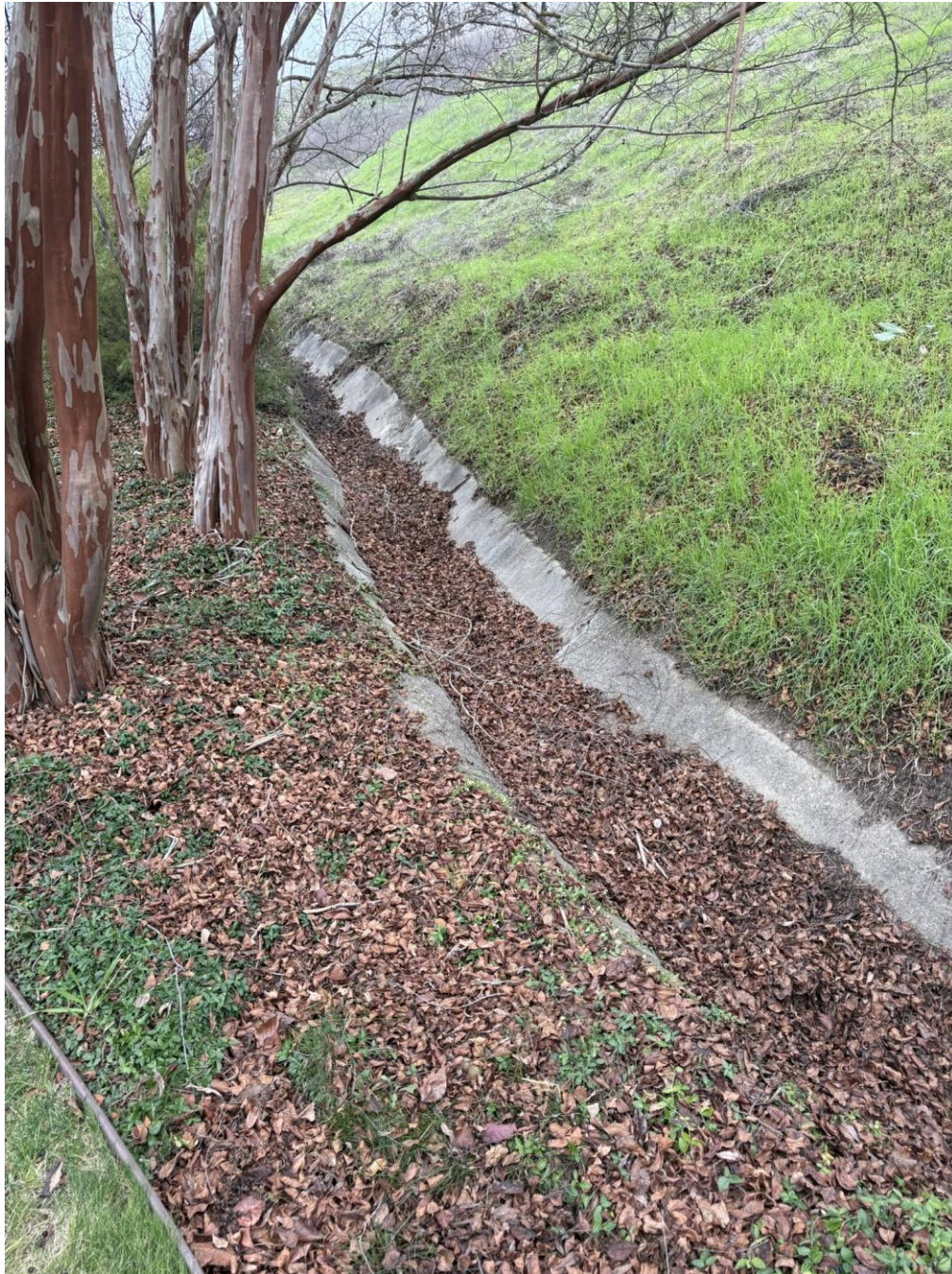
Site Condition C – Photograph 4, Debris in Concrete-Lined Drainage Ditch
