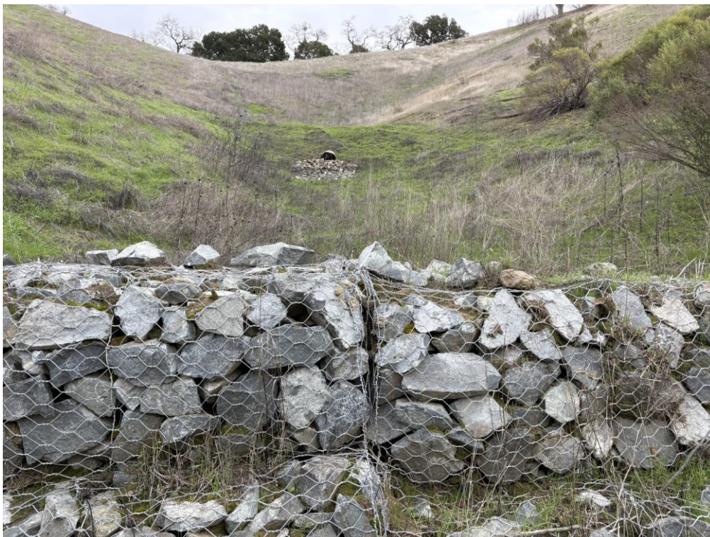
Site Condition E – Photograph 6, MSE Walls and Recent Slope Repairs
