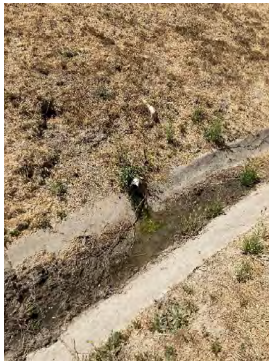
Photo 2. View of subdrain pipe discharging into a concrete-lined v-ditch.
