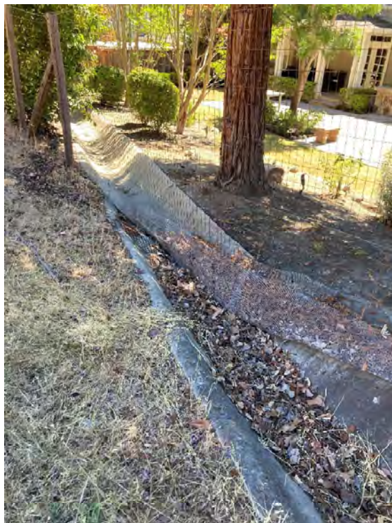
Photo 32. View of fencing extending to v-ditch and blocking debris.
