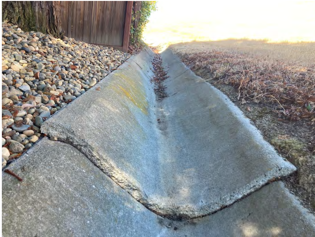
Photo 20. View of a vertical offset of a v-ditch.
