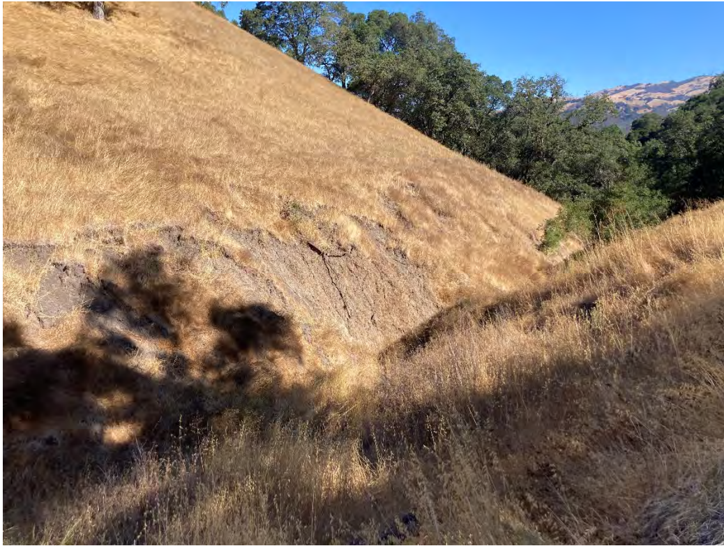
Photo 15. View of the significant erosion in the drainage channel south of 138 Windover Dr.
