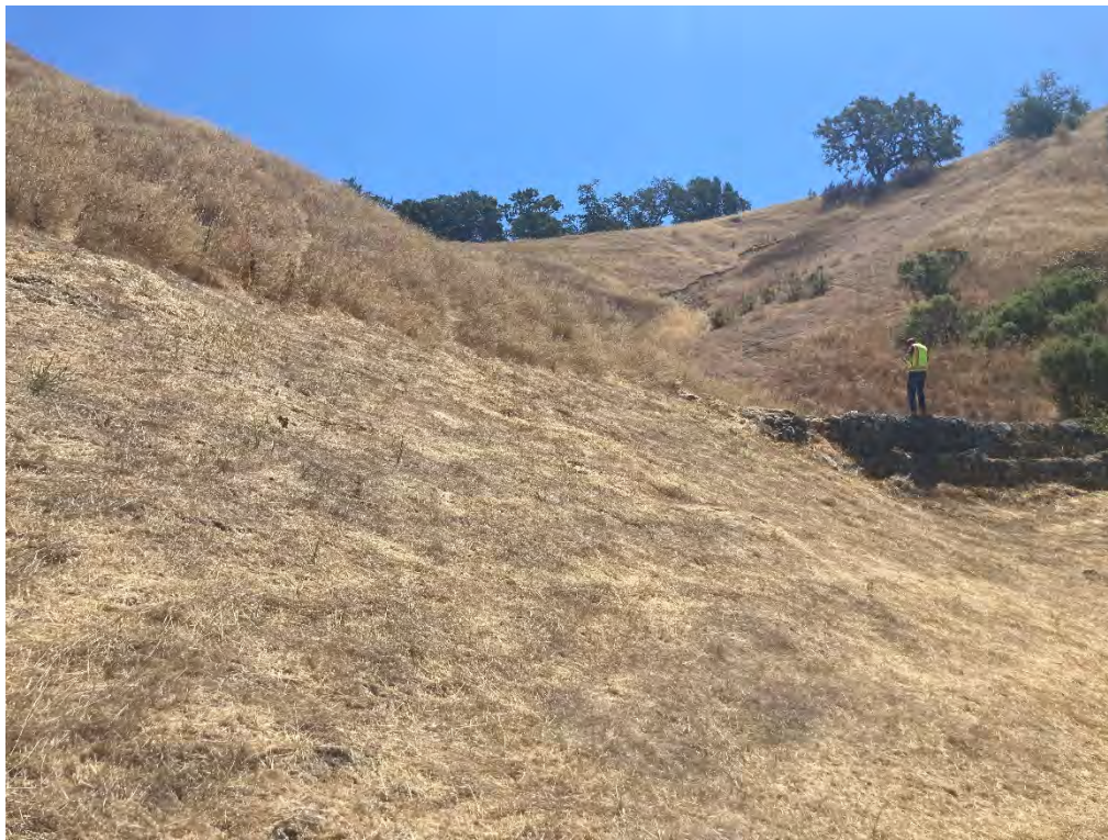
Photo 8. View of recently active landsliding behind 124 Shadewell Drive.
