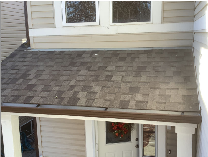
Lower Front Roof
