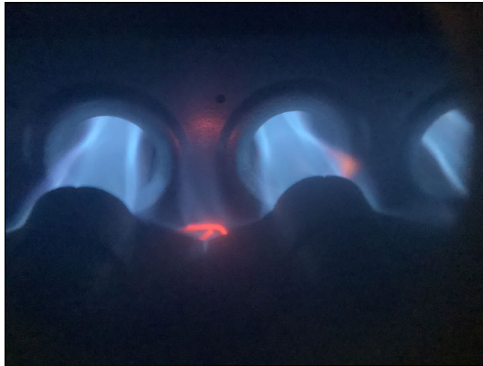
All visibly good in burner chamber on day of inspection
