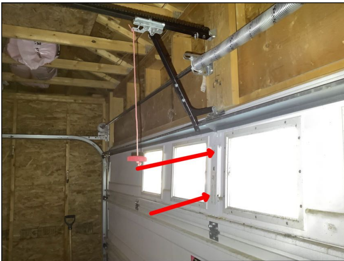
Door bracket is usually attached as shown
