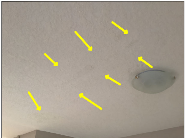
Stains show as dry after running water above
