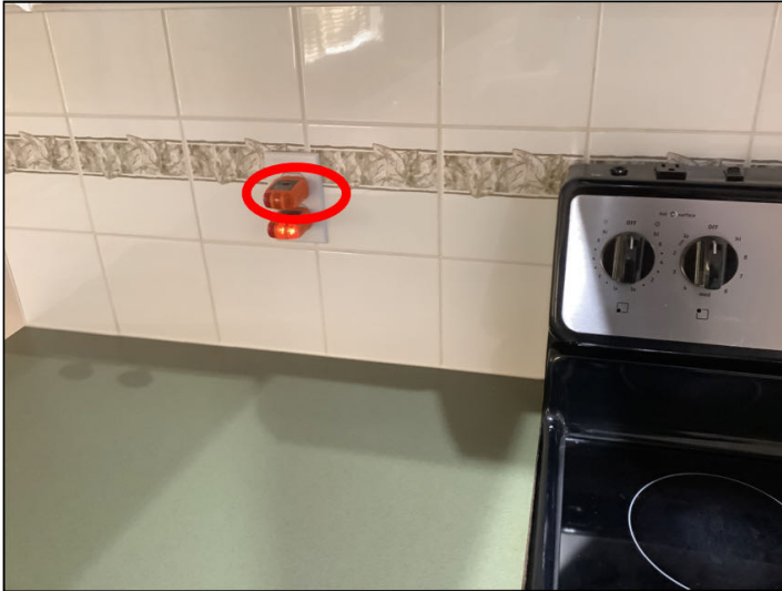
Left of stove - Top receptacle has no power
