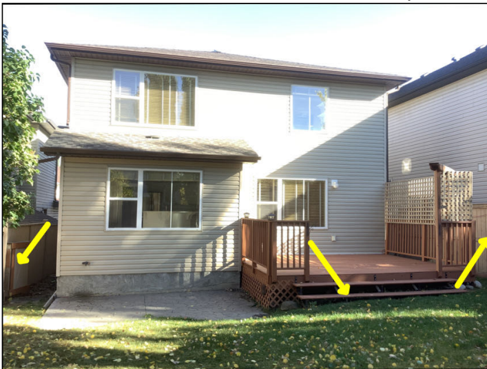
All external wood requires regular maintenance
