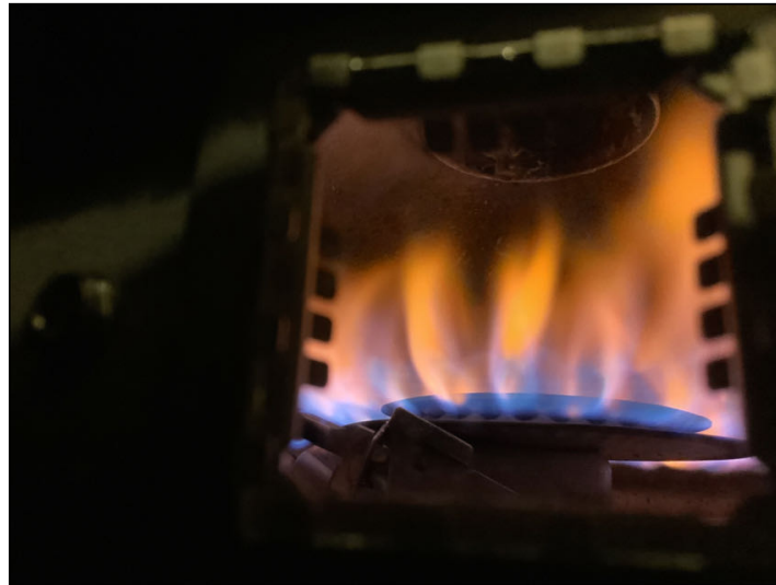
The combustion chamber appears to be in good condition.
