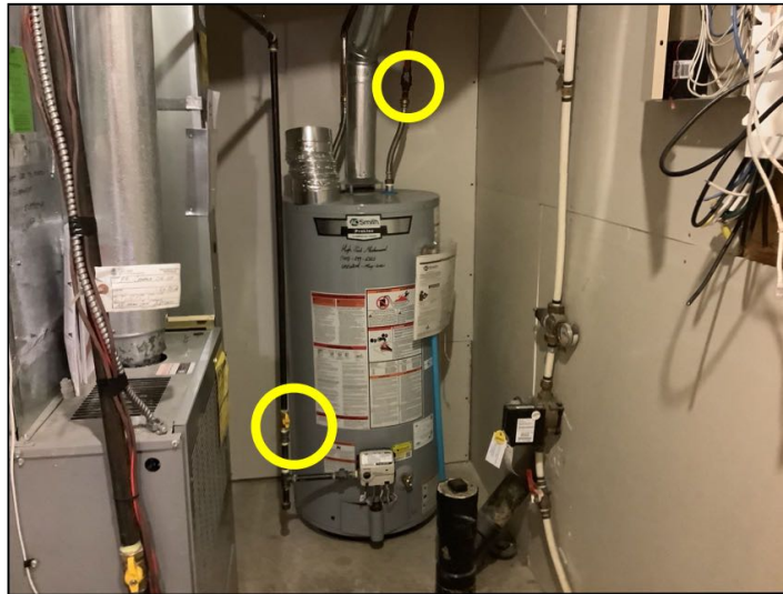
Water and gas shut offs shown.
