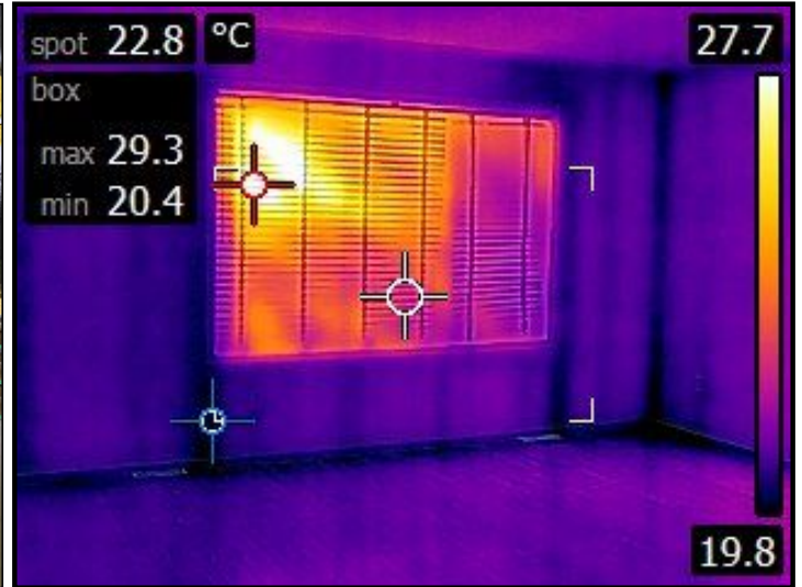
Primary Bedroom - Thermal Image
