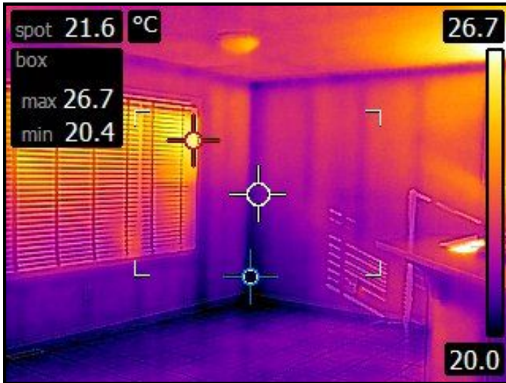
Dining Area - Thermal Image
