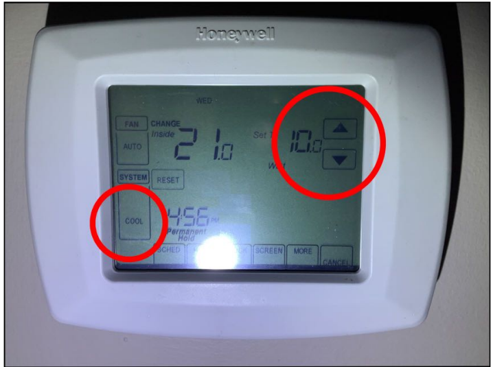
Air conditioning failed to operate using normal controls
