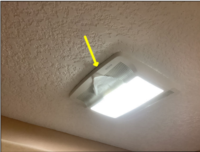
Basement Bathroom- tested and working as required
