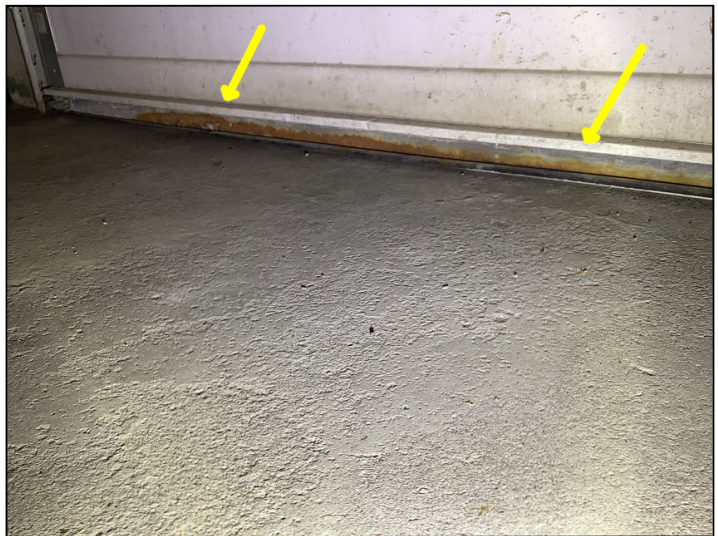
Garage door is rusting at the bottom
