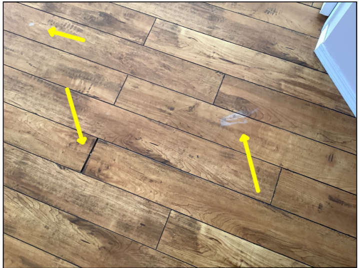
Flooring appears to be in serviceable condition - minor cosmetic issues noted
