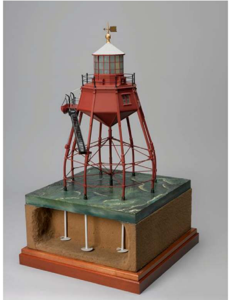
Above: A handmade model of the Maplin Sands Lighthouse, showing a cutaway view of the helical pile foundation.
