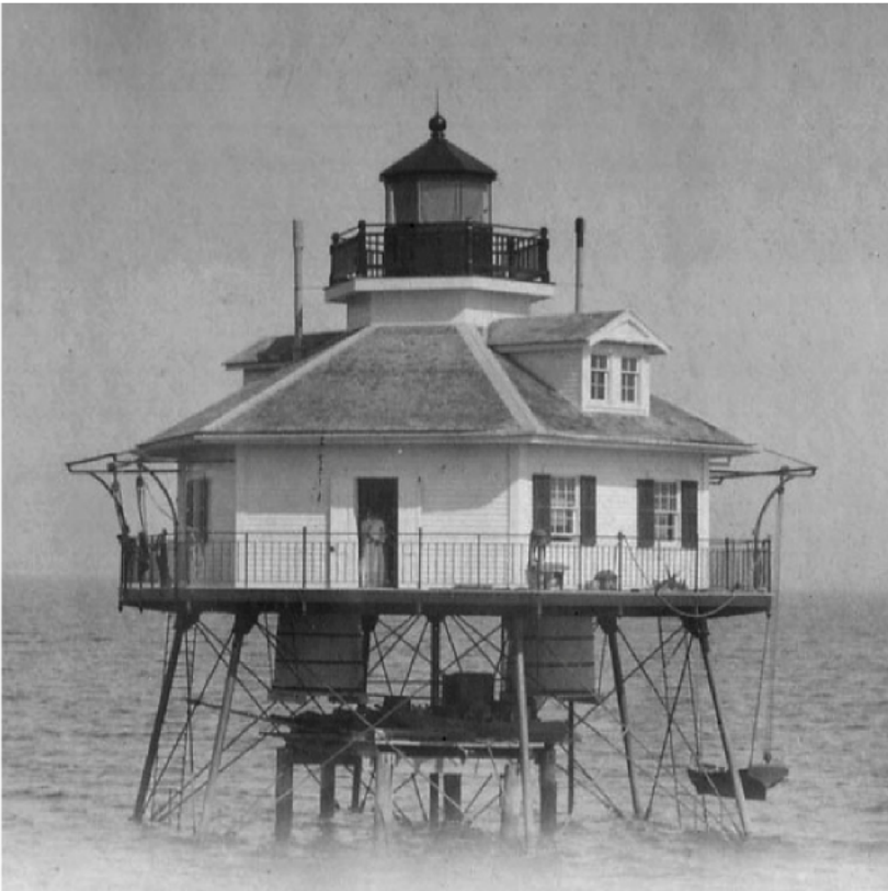
Middle Bay Lighthouse near Mobile, Alabama. Constructed 1885 on helical piles.
