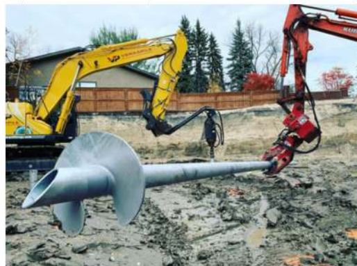
A tractor trailer transported these high-capacity helical piles. Smaller piles can be hauled by a heavy-duty
