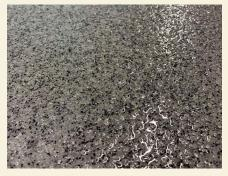
This is an industrial version of our standard SB Quartz Floor. We start with preparing the floor surface by grinding and repairing any damage to the concrete.
