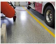
Our SB Flake Floor for Fire Departments is very popular in Atlantic Canada. This is an industrial version of our standard SB Flake Floor. We start with preparing the floor surface by grinding and repairing any damage to the concrete.
