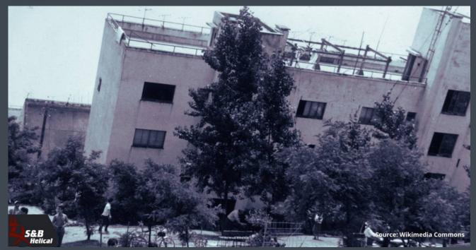
Widespread soil liquefaction during the 1964 earthquake in Niigata, Japan, caused enormous damage to buildings such as these large residential structures that suffered foundation failure
