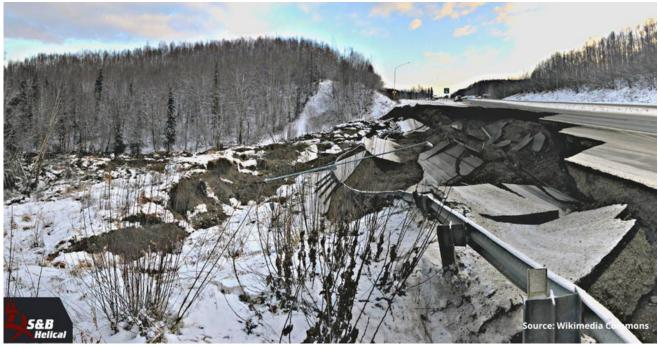
*In the 2018 Alaska earthquake, highways such as the one pictured here suffered severe damage from seismic forces and soil liquefaction*
