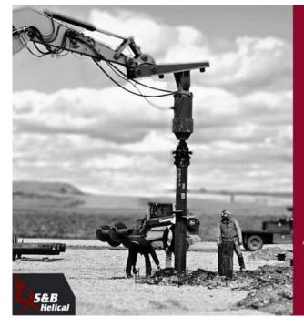
"The use of helical piles resulted in almost no measured differential settlement and tilt of the foundation."
