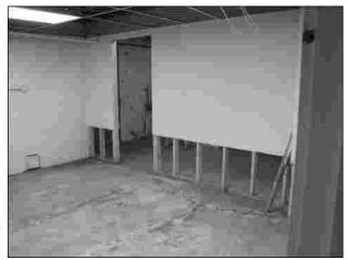
Hence a delayed opening to the Market Pantry. Reconstruction in November of a few walls, new carpeting and ceiling tiles and fresh paint followed the mold removal.
