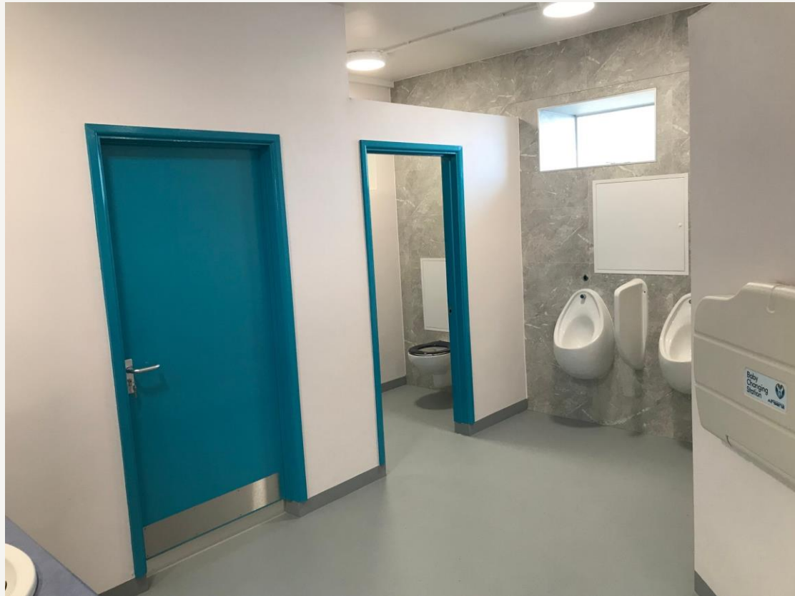
THE REFURBISHED TOILETS AT QUAY WEST CAR PARK.
