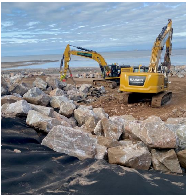
Machinery placing rock along the shingle ridge
