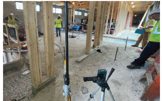
FillFoam™ Pipes Installed
