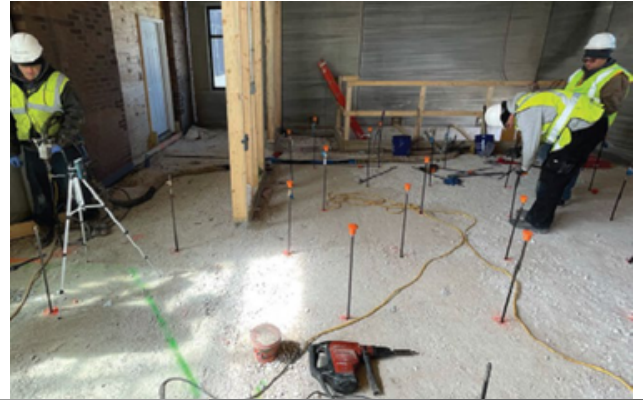
Deep Foamjection™ Pipes Installed
