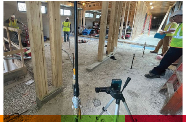
FillFoam™ Pipes Installed
