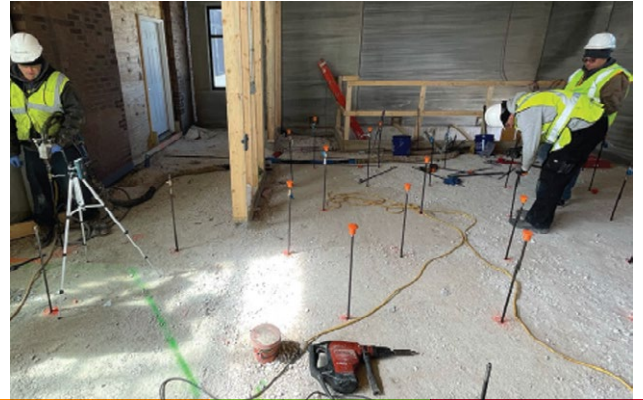
Deep Foamjection™ Pipes Installed
